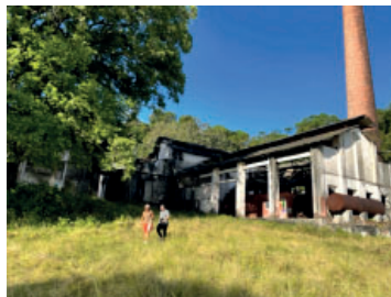
Figure 18: Site of abandoned gunpowder factory
